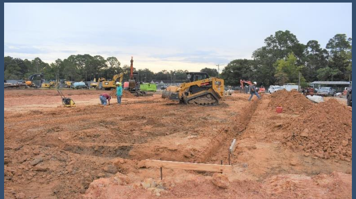
Pool House footers being dug
