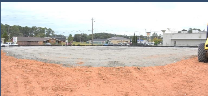
Foundation is being laid for Miracle Field flooring.
