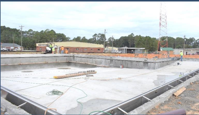
8-lane swimming pool
