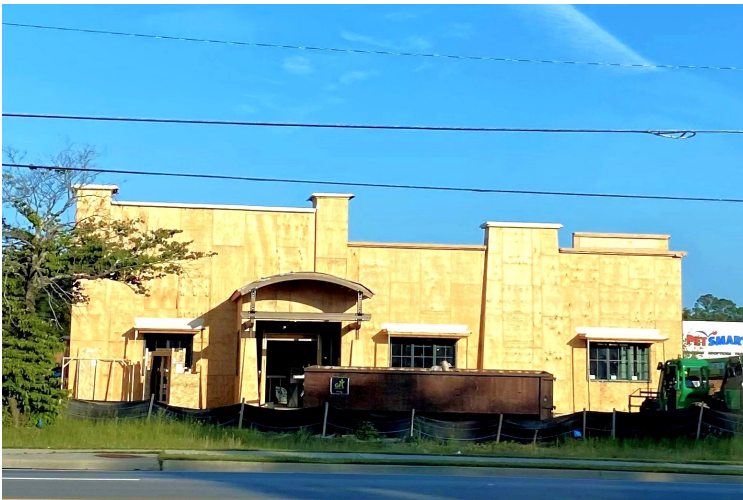
Longhorn construction continues and is moving along at a great pace!
