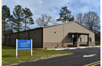
CDBG'2020 funding assisted with the construction of the Coffee County Unison Adult Behavioral Health Services Facility.
