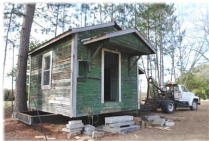
Office being placed on trailer to be moved to new location across from Museum.
