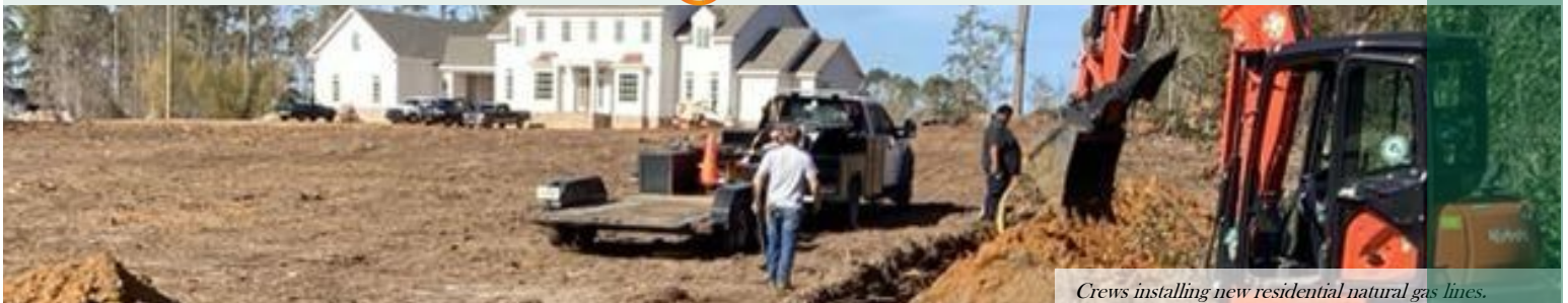
Crews installing new residential natural gas lines.
