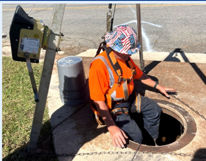
Confined space storm drain repair on Cherry Street.
