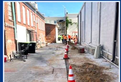
Repair of sewer line in Downtown Douglas
