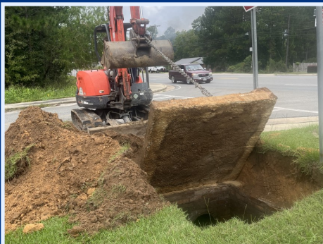
Storm Drain Repair on Hwy 32 & Olliff
