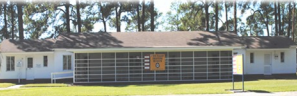
11. Barracks 7—Housing for cadets. Current and Future Usage: WWII Flight Training Museum
